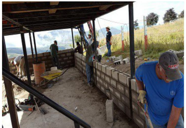
Block by block the wall goes up.
