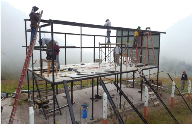
Sheet metal walls going up.
