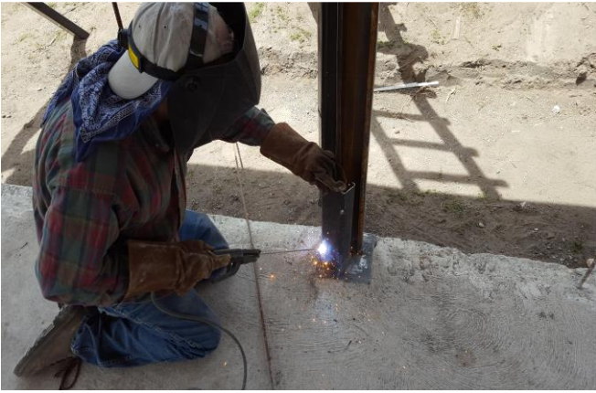
Welding in the support braces.
