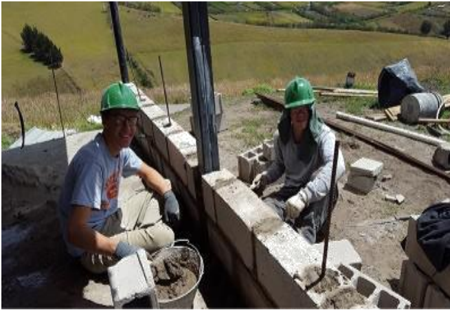
Noah and Sam Galuk filling in mortar.
