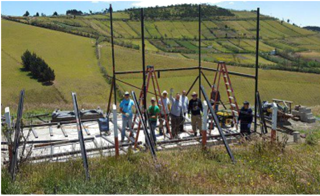
Framework going up.
