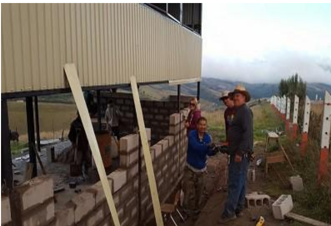
Security wall is almost complete.
